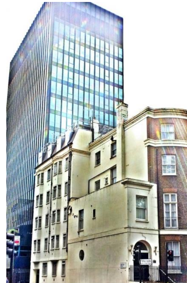
Olallo House TB Hostel
