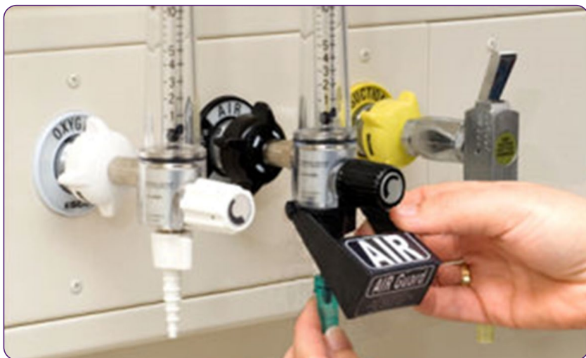
Figure 1 AIR FLOWMETER WITH MOVEABLE FLAP
